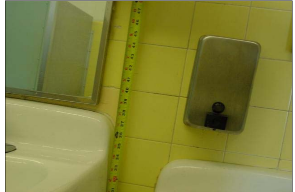
Boys Restroom Building A
