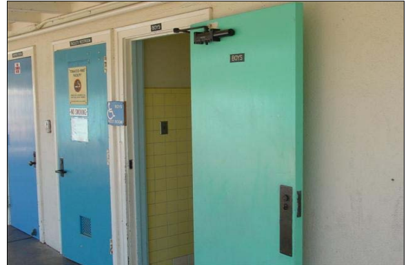
Boys Restroom Building A
