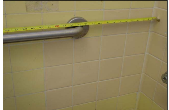
Boys Restroom Building A
