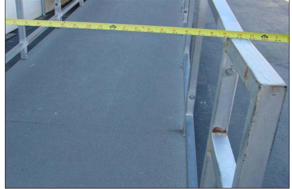
Ramp to Rooms 37 and 38
