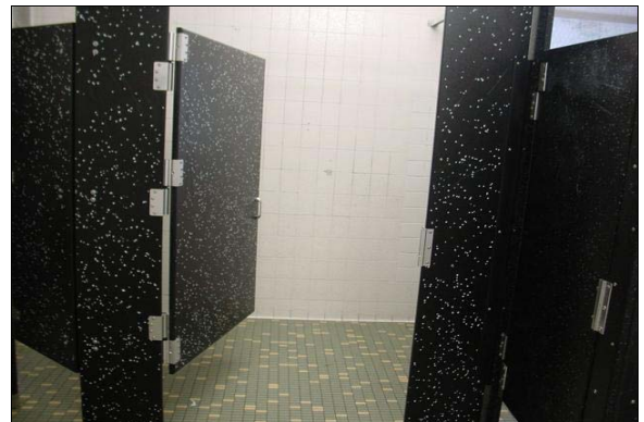
Boys Restroom Building M
