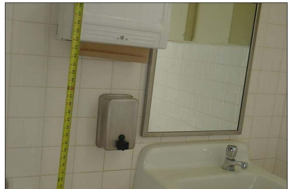
Unisex Restroom in Shop Building Room 62
