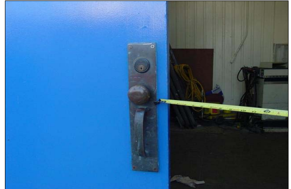
Accessible Route to the Home Economics Restrooms
