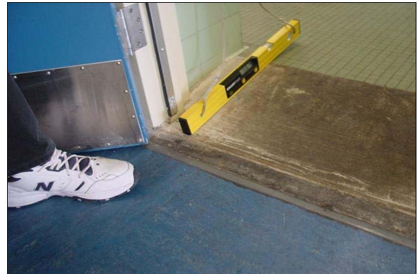
Boys Restroom Across from Room 33 Admin. Building
