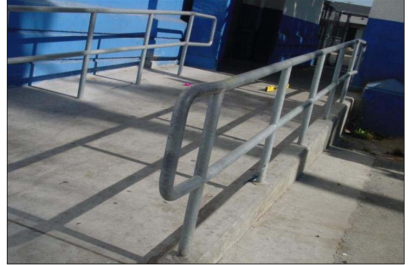
Accessible Route to the Cafeteria
