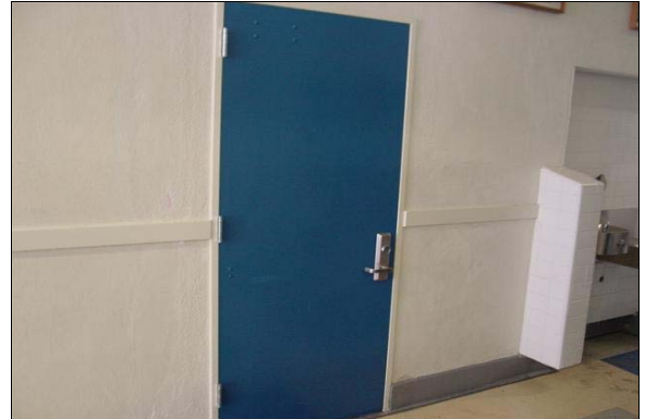
Girls Restroom Across from Room 25 Admin. Building
