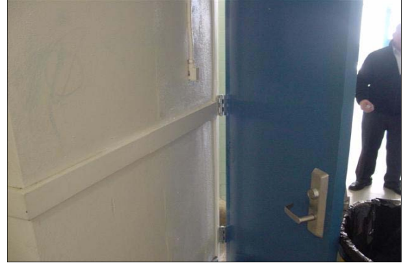
Boys Restroom Across from Room 33 Admin. Building
