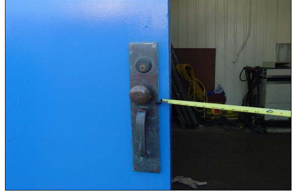
Accessible Route to the Home Economics Restrooms
