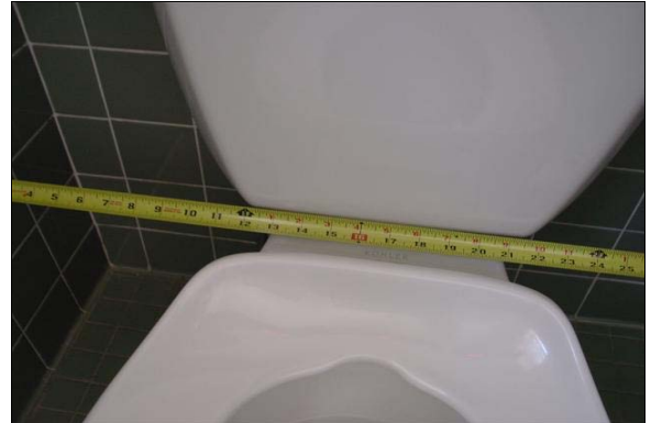
Staff Unisex Restroom Second Floor Administration Building
