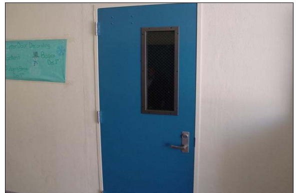
Staff Unisex Restroom Second Floor Administration Building
