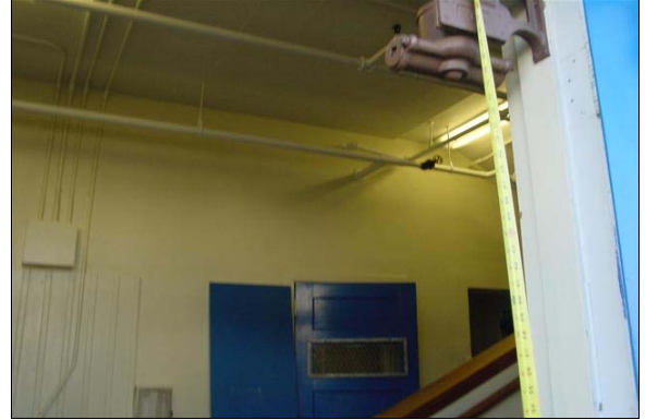
Accessible Route to the Home Economics Restrooms
