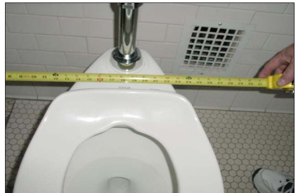
Girls Restroom first floor Home Economics Bldg.
