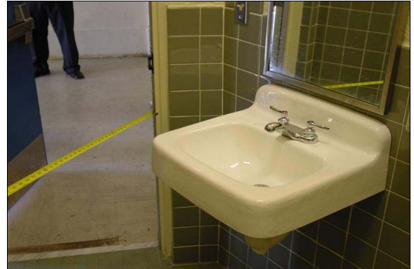
Staff Mens Restroom First Floor Administration Building
