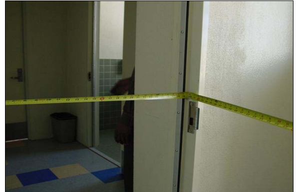
Staff Unisex Restroom Second Floor Administration Building
