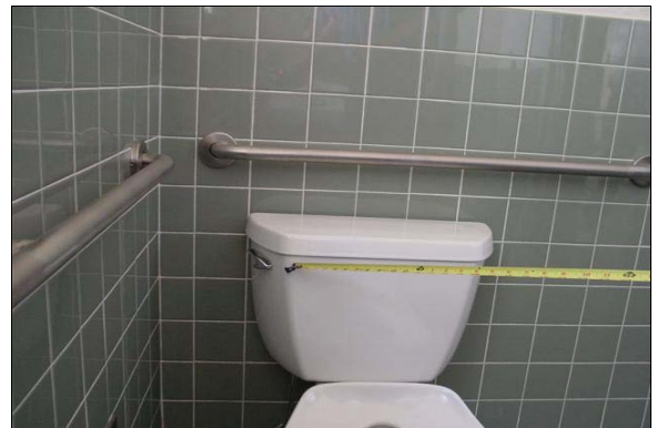
Staff Unisex Restroom Second Floor Administration Building
