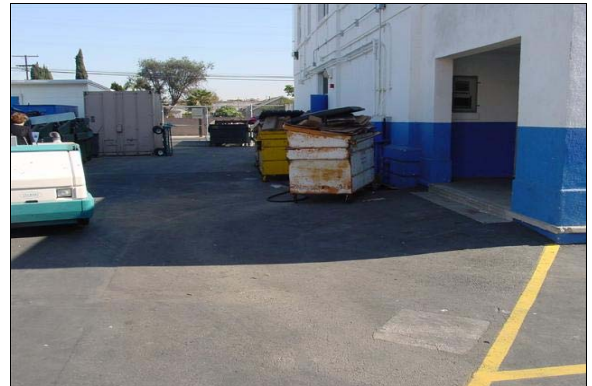
Accessible Route to the Home Economics Restrooms
