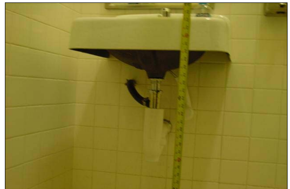
Unisex Restroom in Shop Building Room 61
