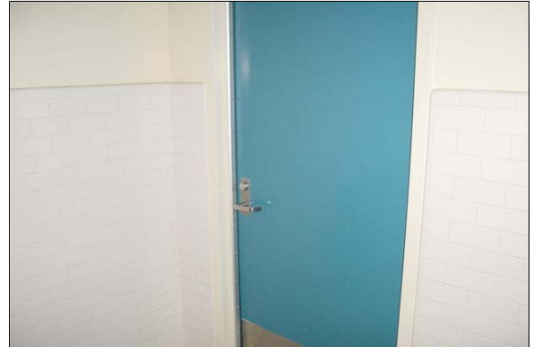
Girls Restroom first floor Home Economics Bldg.
