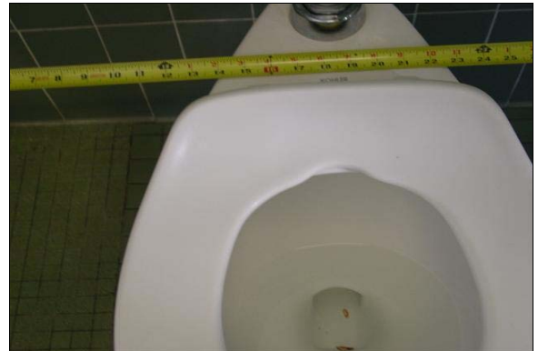
Boys Restroom Across from Room 33 Admin. Building
