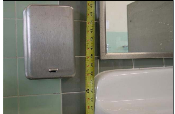
Boys Restroom Across from Room 33 Admin. Building
