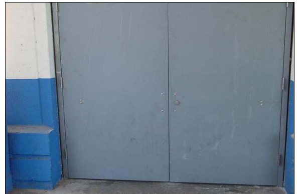
Accessible Route to the Cafeteria
