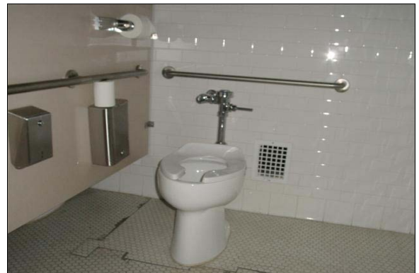
Girls Restroom first floor Home Economics Bldg.
