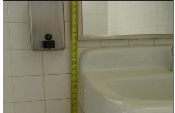
Unisex Restroom in Shop Building Room 62
