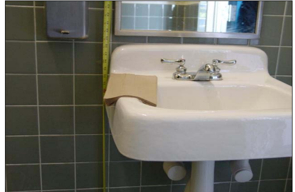
Staff Womens Restroom First Floor Administration Building
