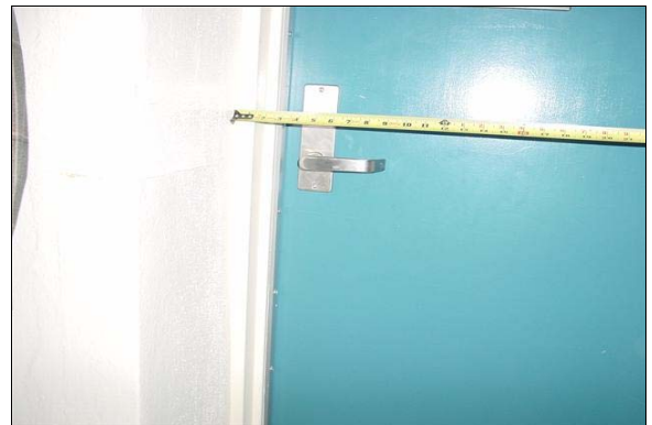
Staff Unisex Restroom Second Floor Administration Building
