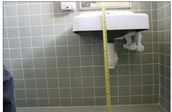
Staff Unisex Restroom Second Floor Administration Building
