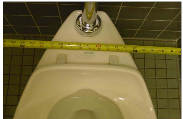
Staff Mens Restroom First Floor Administration Building
