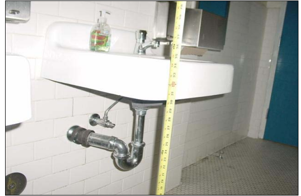
Girls Restroom first floor Home Economics Bldg.
