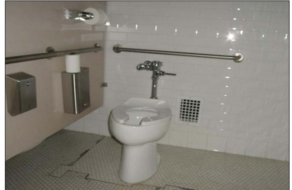
Girls Restroom first floor Home Economics Bldg.
