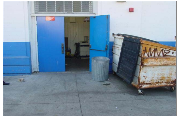
Accessible Route to the Home Economics Restrooms
