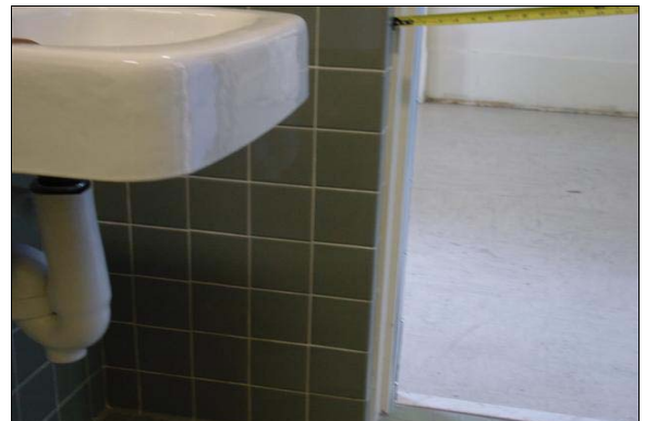
Staff Womens Restroom First Floor Administration Building
