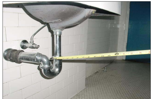
Girls Restroom first floor Home Economics Bldg.
