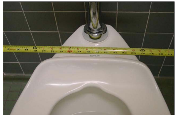
Staff Womens Restroom First Floor Administration Building
