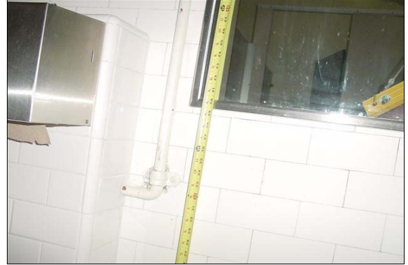
Girls Restroom first floor Home Economics Bldg.
