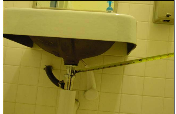
Unisex Restroom in Shop Building Room 61
