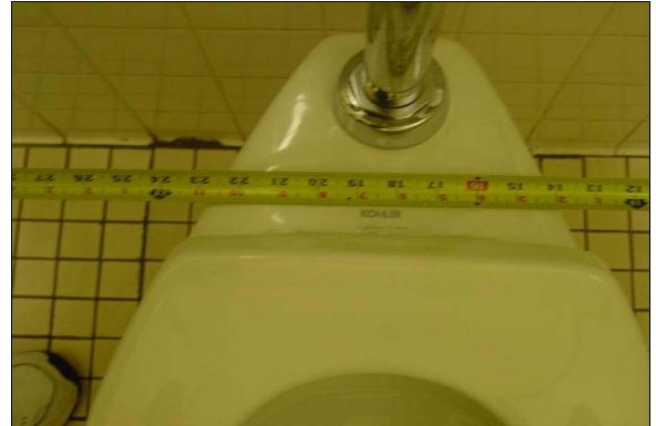
Unisex Restroom in Shop Building Room 61
