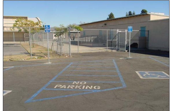
Accessible Parking Next to Room B6
