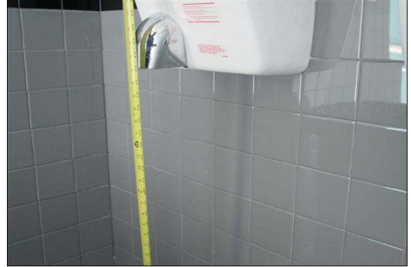
Girls Restroom Next to Room 65
