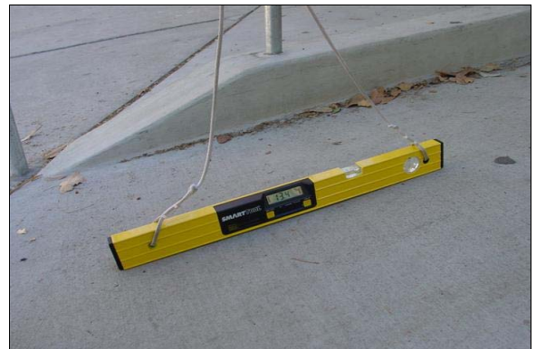
Ramp to Nurse Office
