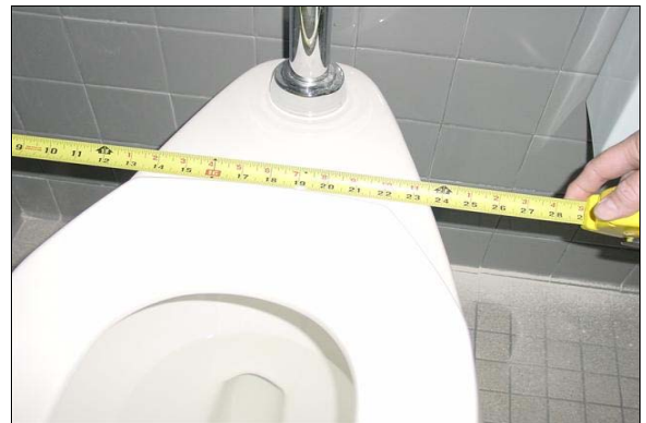
Girls Restroom Next to Room 65
