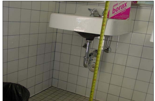
Womens Staff Restroom Next to Room 65
