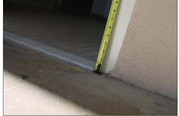
Womens Staff Restroom Next to Room 65
