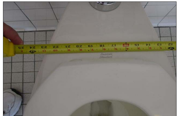
Womens Staff Restroom Next to Room 65
