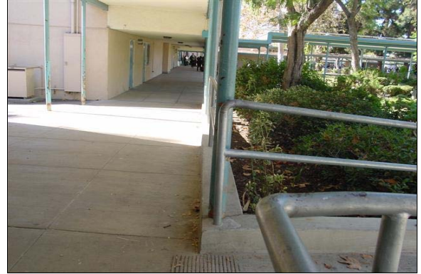
Ramp to Nurse Office
