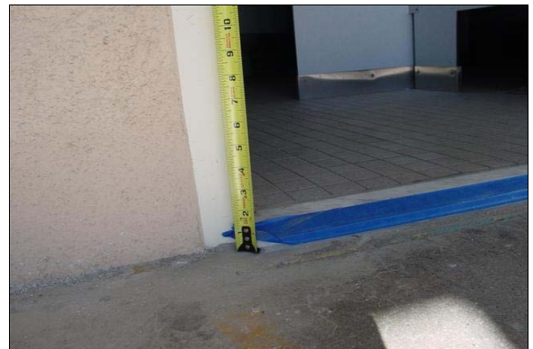
Girls Restroom Next to Room 65
