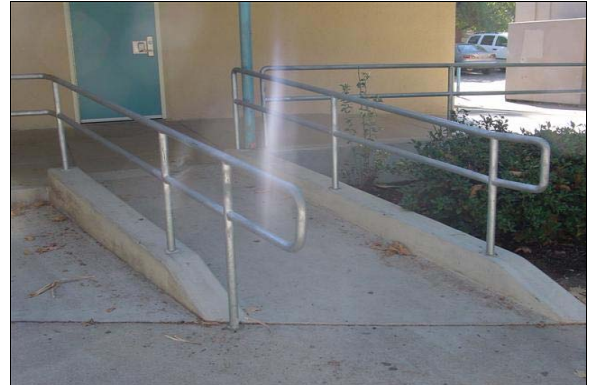
Ramp to Nurse Office
