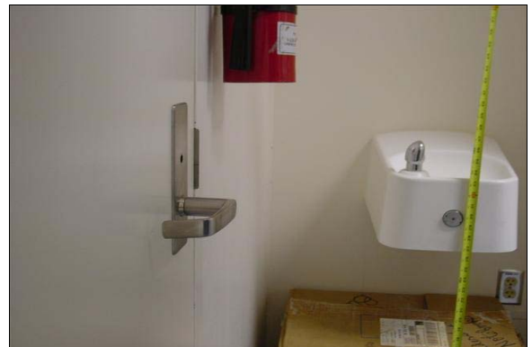
Drinking Fountain Next to the Assistant Principals Office
