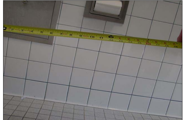
Womens Staff Restroom Next to Room 65
