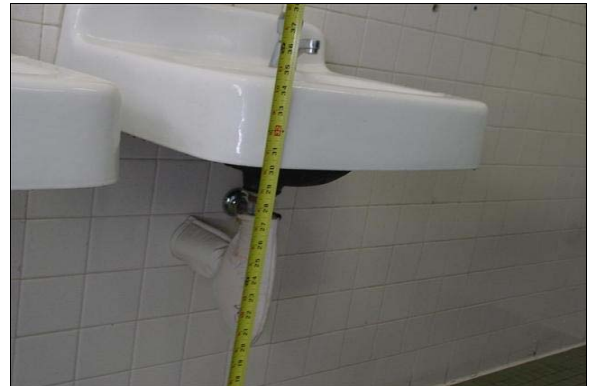
Boys Restroom Building E
