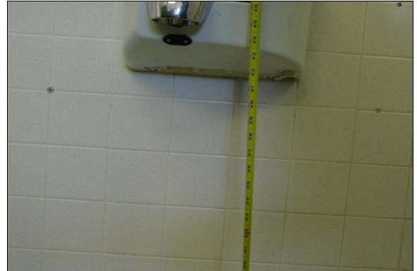
Boys Restroom Building E
