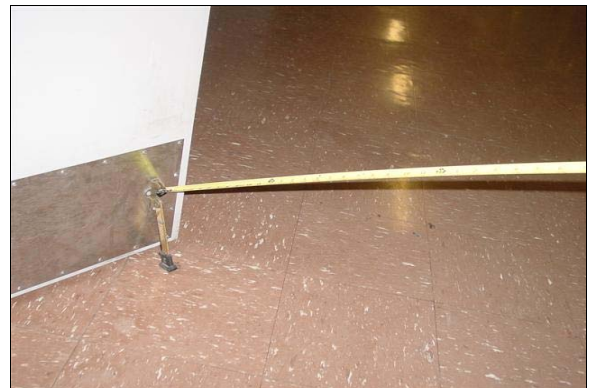
Boys Restroom Building C
