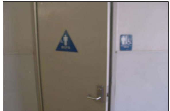
Boys Restroom Building F
