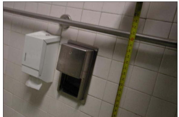
Boys Restroom Building B
