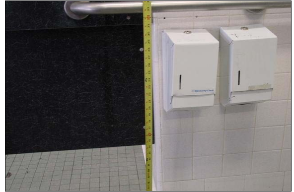
Boys Restroom Building E
