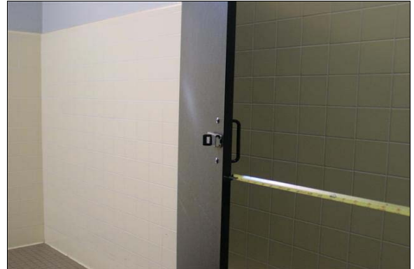
Girls Restroom Building C
