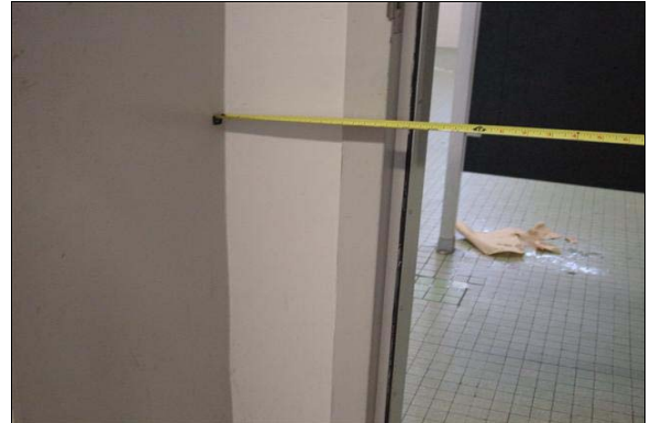
Boys Restroom Building C
