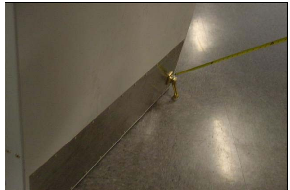
Boys Restroom Building B
