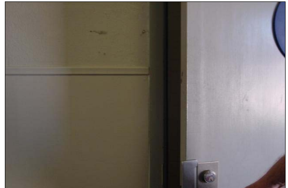
Girls Restroom Building B
