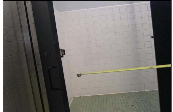
Boys Restroom Building C
