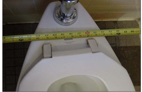
Girls Restroom Building B
