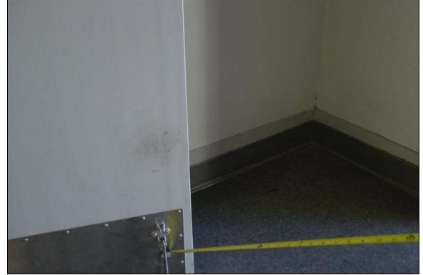
Girls Restroom Building B
