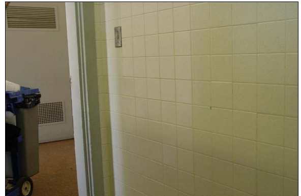
Boys Restroom Building E
