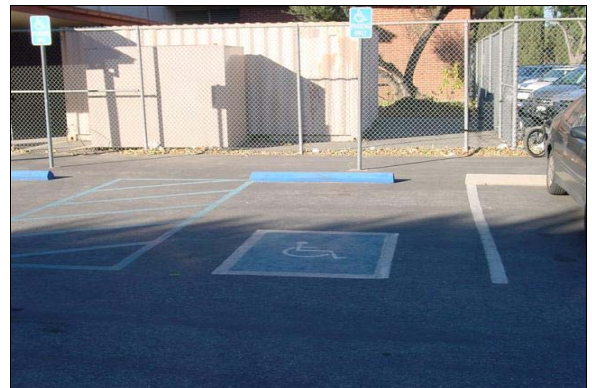
Accessible Parking Next to Multi-Purpose Room
