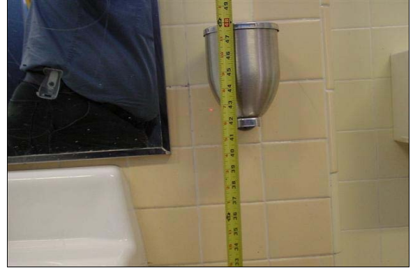
Girls Restroom Building B
