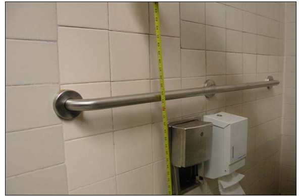
Boys Restroom Building T
