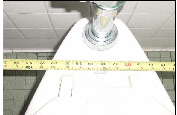
Boys Restroom Building B
