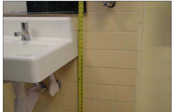
Girls Restroom Building B
