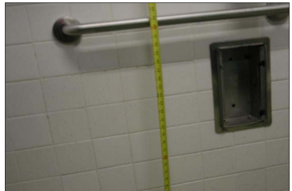
Boys Restroom Building F
