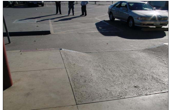
Curb Ramp at Passenger Loading Zone Next to Shop
