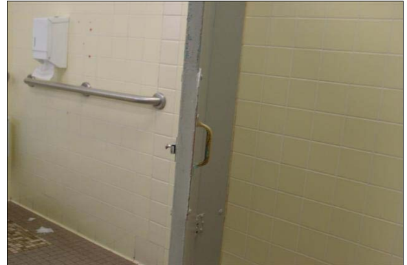
Girls Restroom Building E
