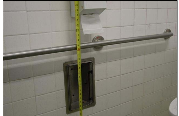
Boys Restroom Building F
