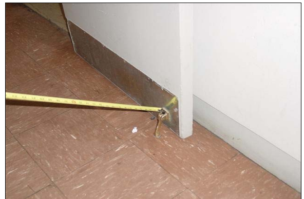
Girls Restroom Building E
