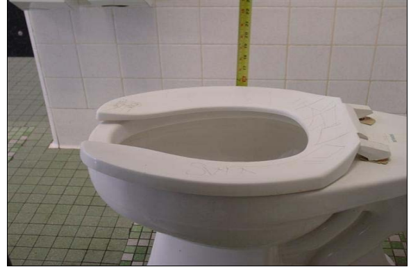
Boys Restroom Building E
