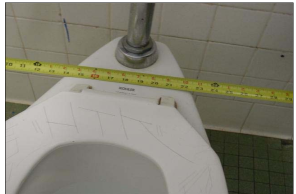
Boys Restroom Building F
