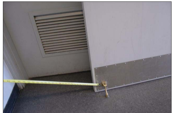
Boys Restroom Building T
