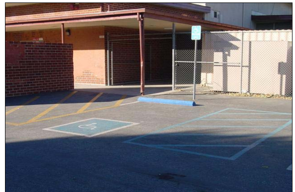
Accessible Parking Next to Multi-Purpose Room
