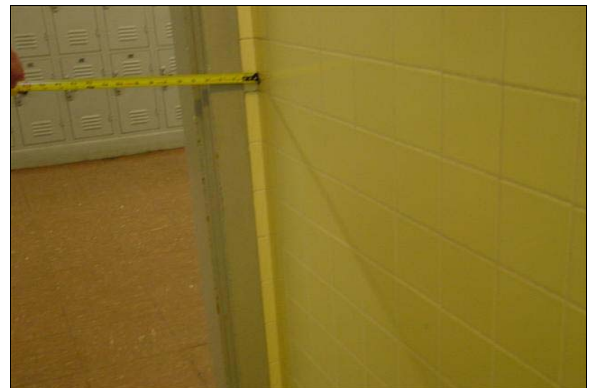
Girls Restroom Building E
