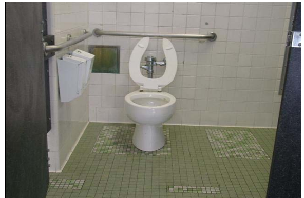
Boys Restroom Building E
