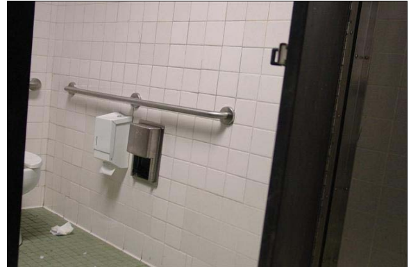
Boys Restroom Building B
