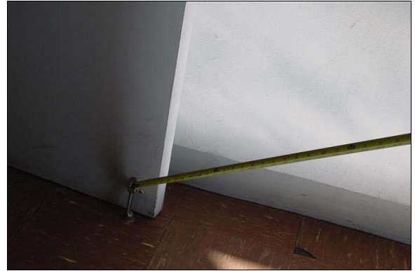
Boys Restroom Building E
