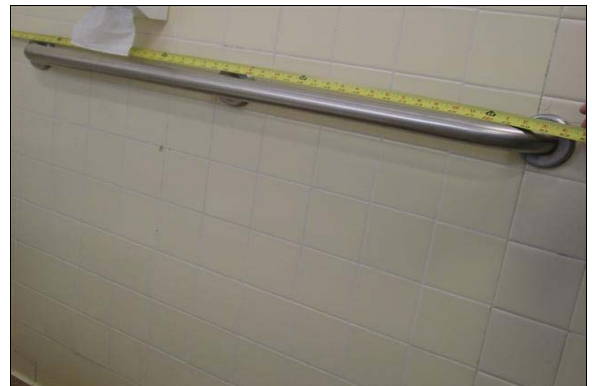
Girls Restroom Building E
