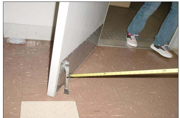
Girls Restroom Building C
