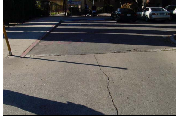
Accessible Parking Next to Main Entrance
