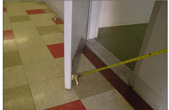
Boys Restroom Building F
