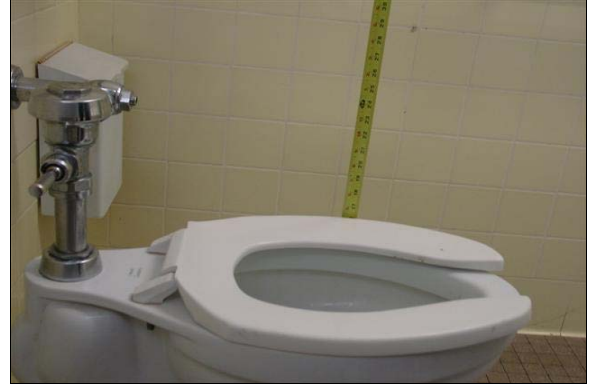
Girls Restroom Building E
