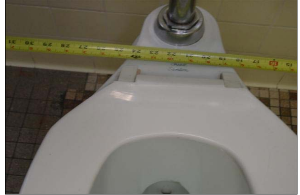
Girls Restroom Building E
