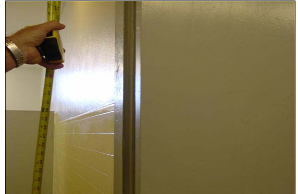
Girls Restroom Building E
