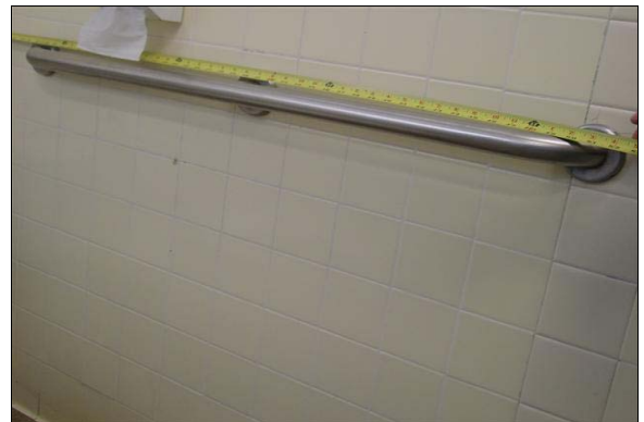
Girls Restroom Building E
