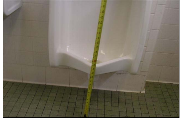
Boys Restroom Building E
