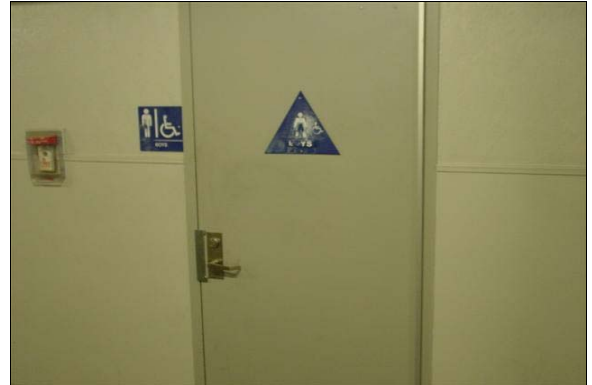
Boys Restroom Building B
