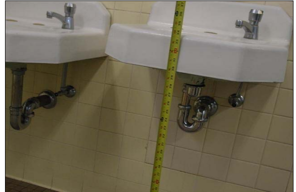
Girls Restroom Building E
