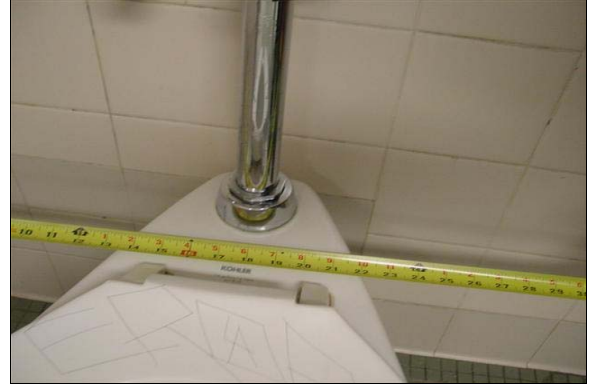
Boys Restroom Building T
