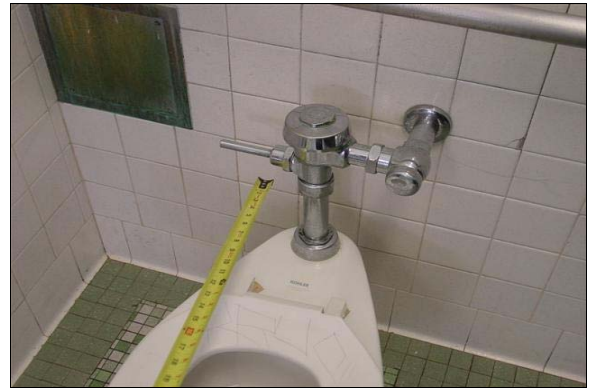
Boys Restroom Building E
