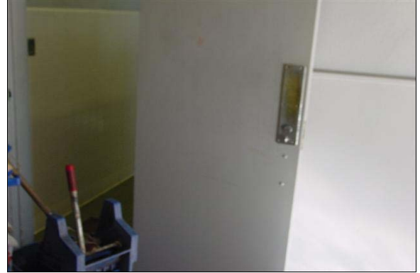
Boys Restroom Building E
