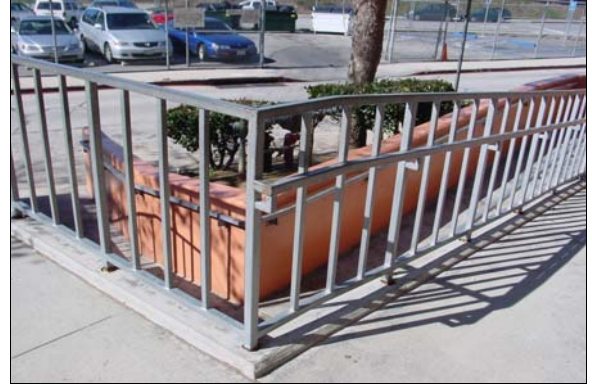
Exterior Ramp at the Main Entrance
