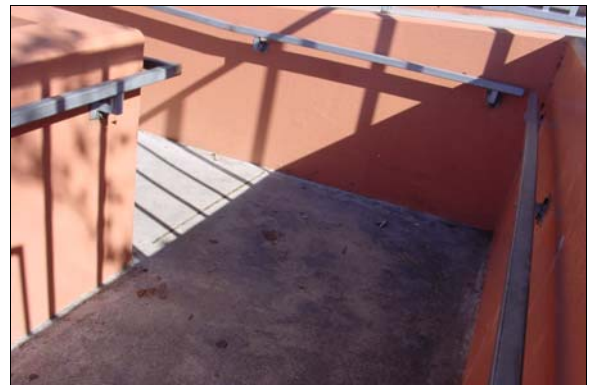
Exterior Ramp at the Main Entrance
