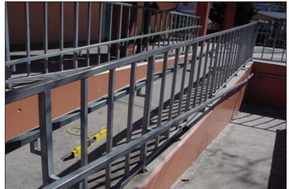
Exterior Ramp at the Main Entrance
