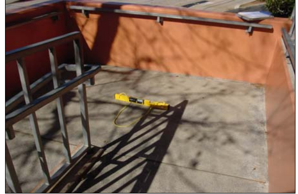
Exterior Ramp at the Main Entrance
