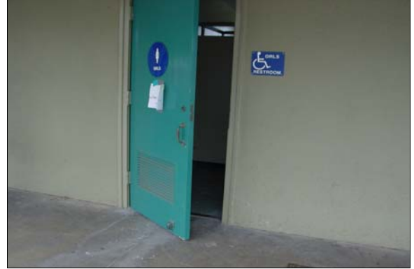
Girls Restroom in Building D
