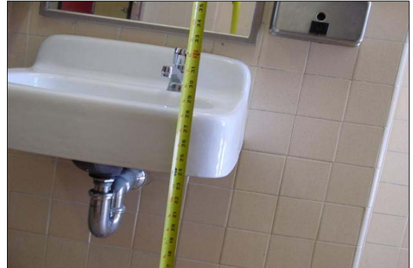
Boys Restroom Next to Room 16
