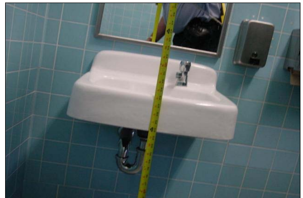
Girls Restroom Next to Room 16
