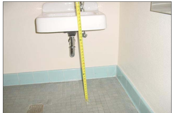
Womens Restroom in Auditorium
