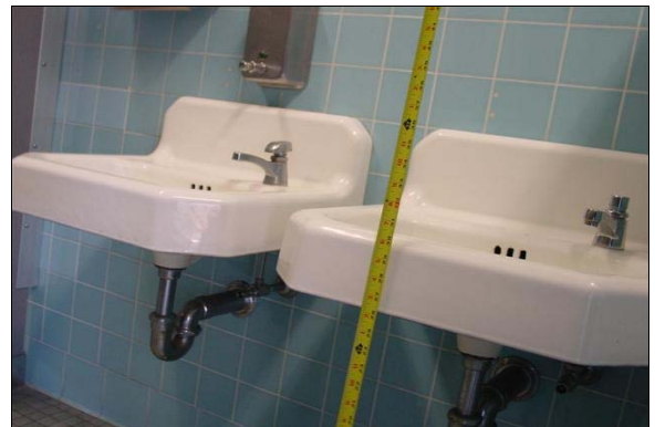
Girls Restroom Next to Room 16
