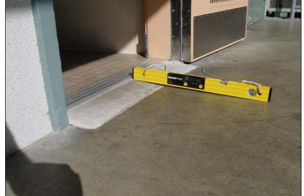
Boys Restroom Next to Room 16
