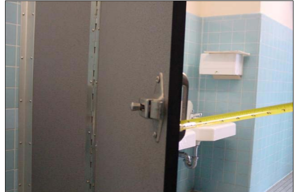
Girls Restroom Next to Room 16
