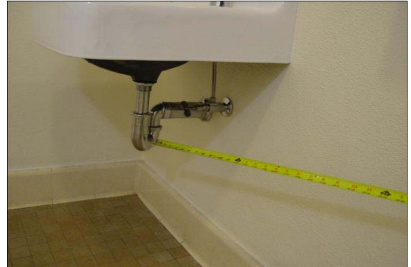
Mens Restroom in Auditorium
