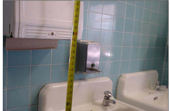
Girls Restroom Next to Room 16
