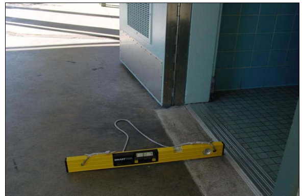
Girls Restroom Next to Room 16
