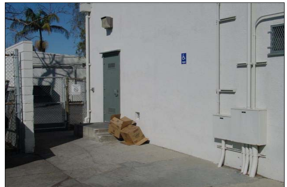
Route to Entrance Gate Next to Auditorium
