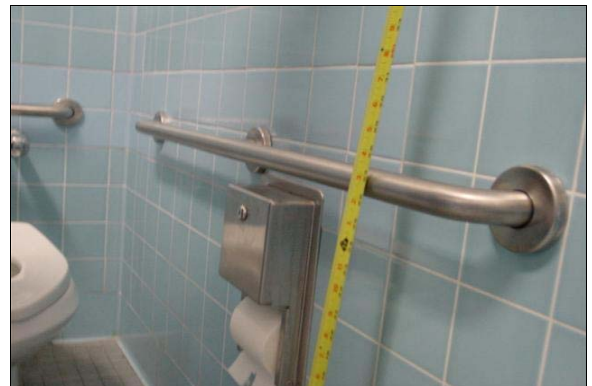
Girls Restroom Next to Room 16
