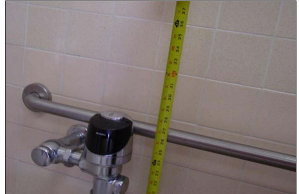
Boys Restroom Next to Room 16
