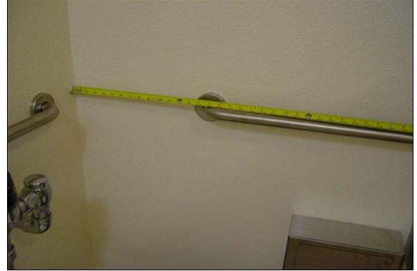
Mens Restroom in Auditorium
