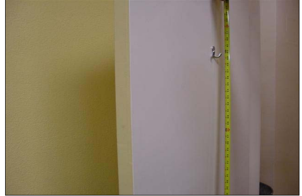
Mens Restroom in Auditorium
