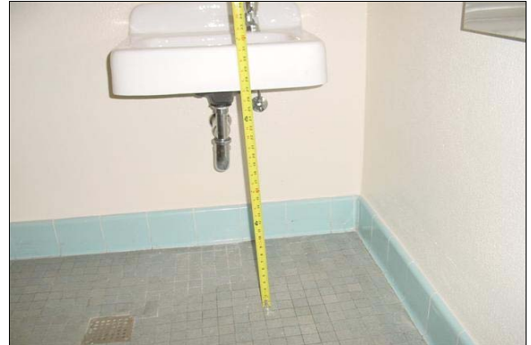
Womens Restroom in Auditorium
