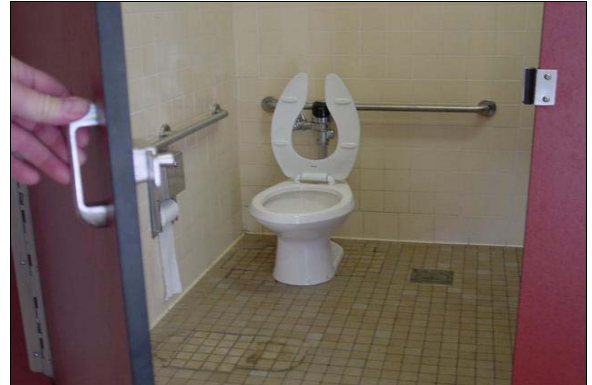
Boys Restroom Next to Room 16
