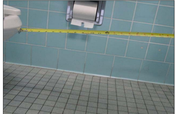
Girls Restroom Next to Room 16
