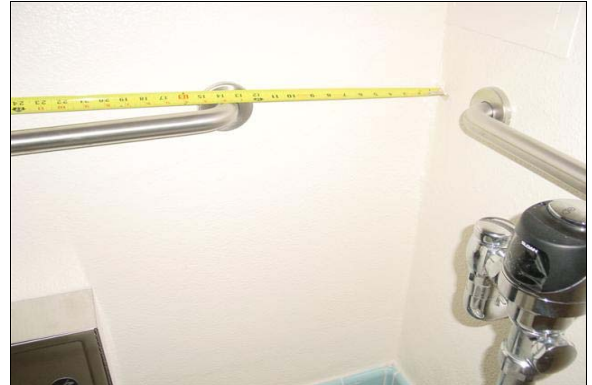
Womens Restroom in Auditorium
