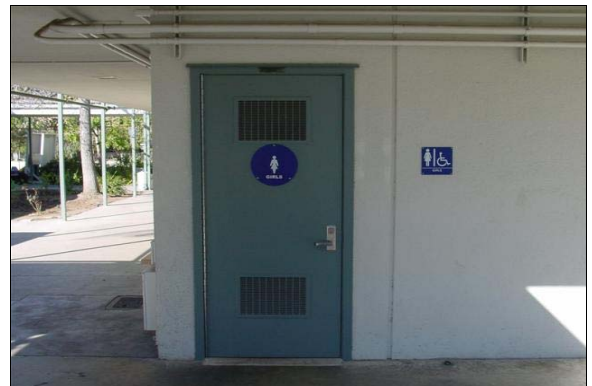
Girls Restroom Next to Room 16
