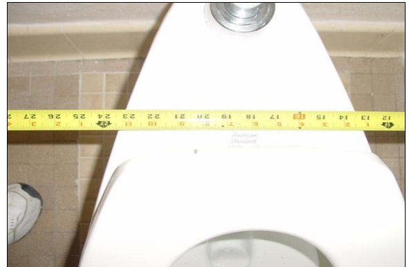
Mens Restroom in Auditorium
