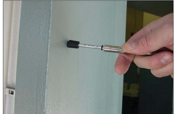
Girls Restroom Next to Room 16
