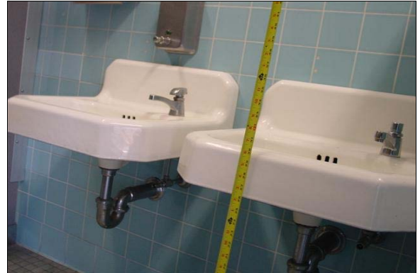
Girls Restroom Next to Room 16
