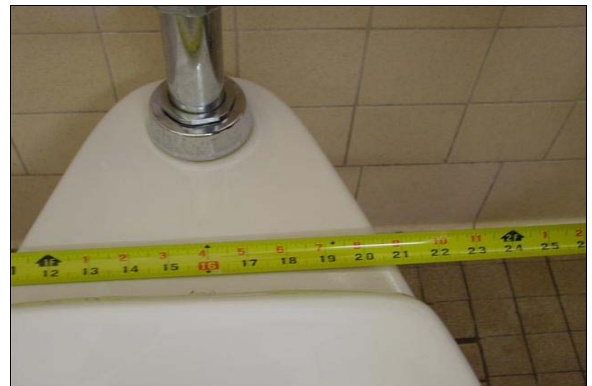
Boys Restroom Next to Room 16
