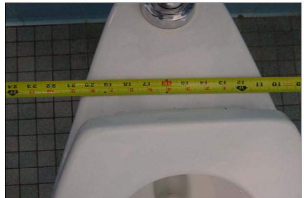
Girls Restroom Next to Room 16
