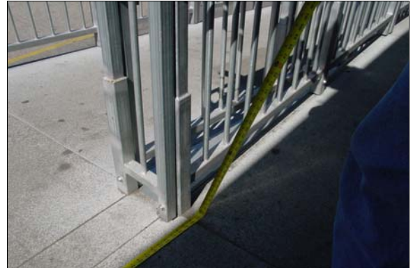
Ramp to Portables 28 & 29
