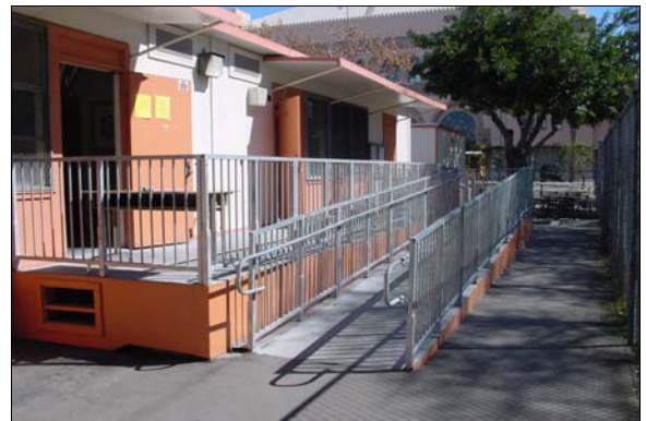
Ramp to Portables 34 & 35
